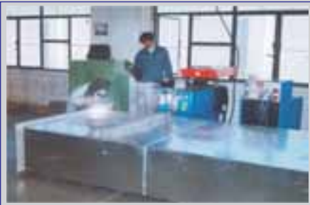
Welding on SPBD
