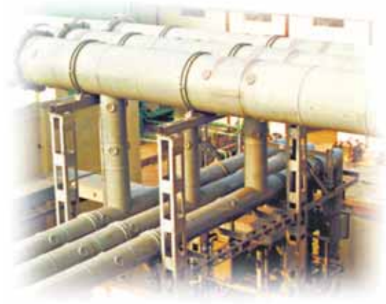
Segregated / Non-Segregated Phase Busduct (415 - 33KV up to 5000 Amps.)
